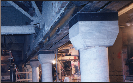
Structural Isolation, Zankel Auditorium, Carnegie Hall
