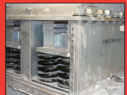
INSTALLATION- Spring Isolators Placed Under Support Columns at NY Times Building NYC
