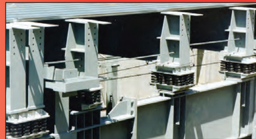
Spring Isolators Close to Rail Lines Supporting the Federation Square Building, Melbourne, Australia
