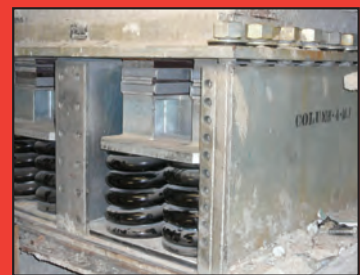
INSTALLATION- Spring Isolators Placed Under Support Columns at NY Times Building NYC
