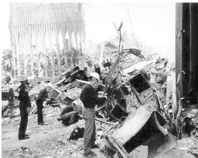
Three members of the Penn State team (hard hats) make background noise measurements at the World Trade Center site. Tom Gabrielson is in the foreground with Matt Poese and Tom Donnellan behind him. At the right is the Bankers Trust Building.
